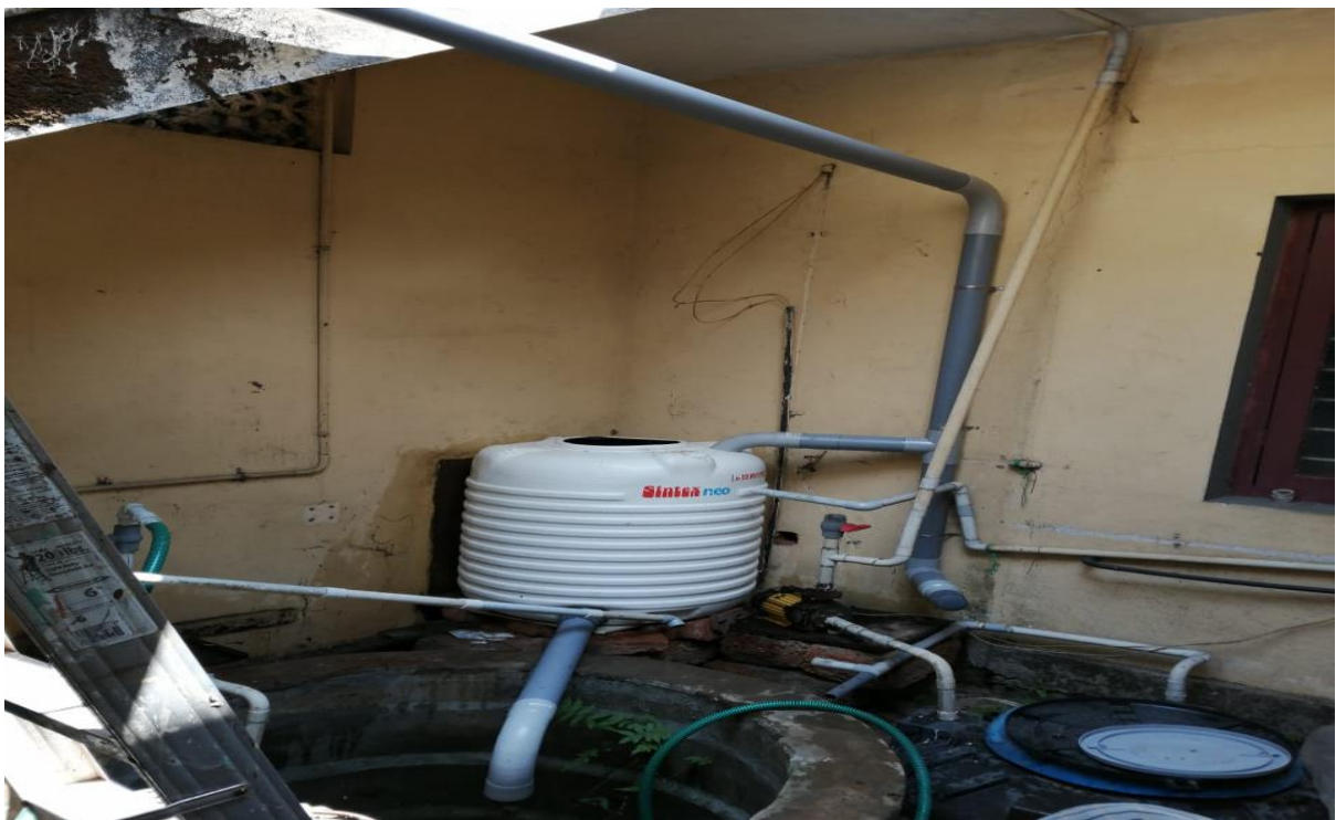
Plate 4. Artificial well recharging technique demonstration plot established under the project at Vytilla, Ernakulam District
