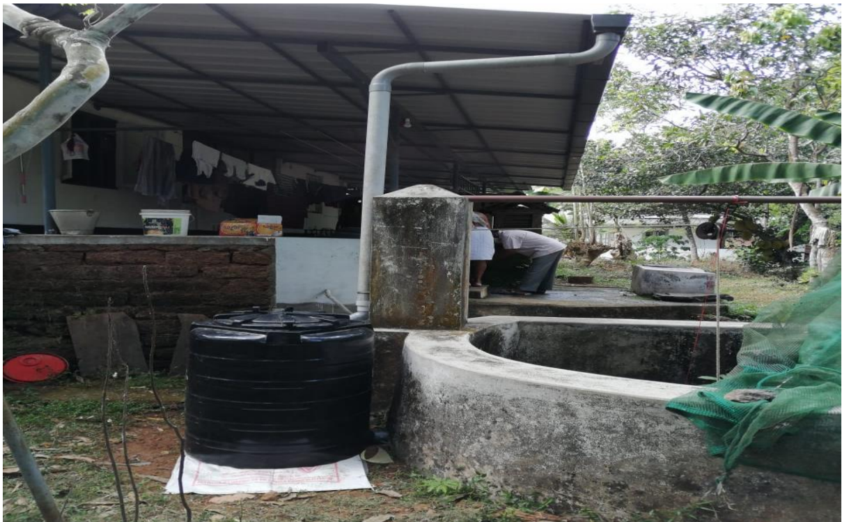
Plate 2. Artificial well recharging technique demonstration plot established under the project at Manjeripadi, Muvattupuzha, Ernakulam District
