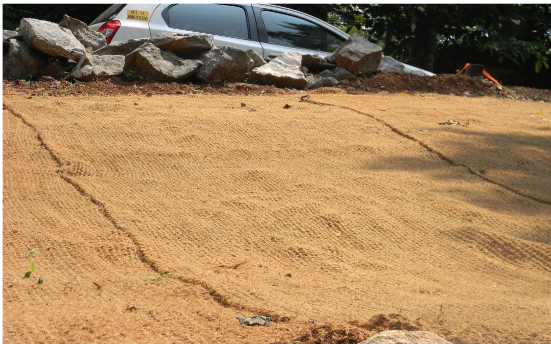
Coir geo-textile laid out as a soil conservation measure in the demonstration plot
