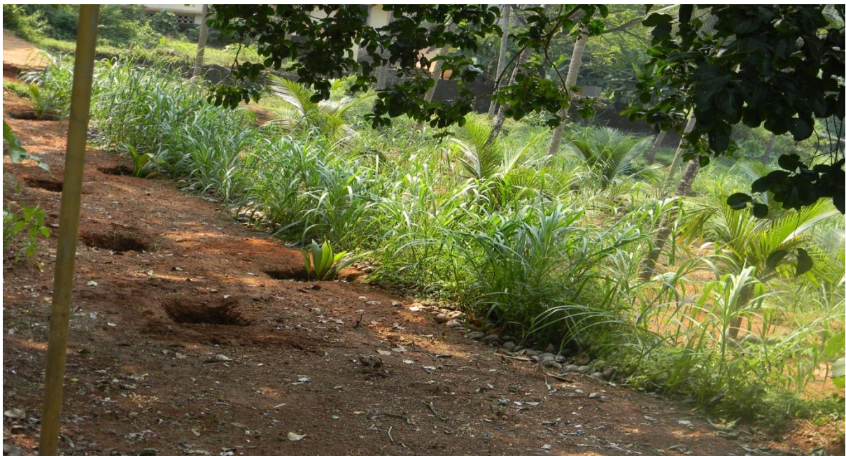
Silt pit in the demonstration plot for ground water recharge
