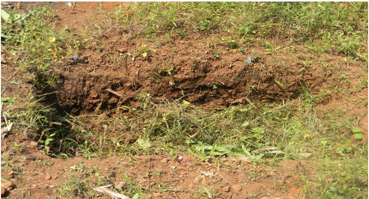
Pate14. Rectangular pit for ground water recharge in the demonstration plot
