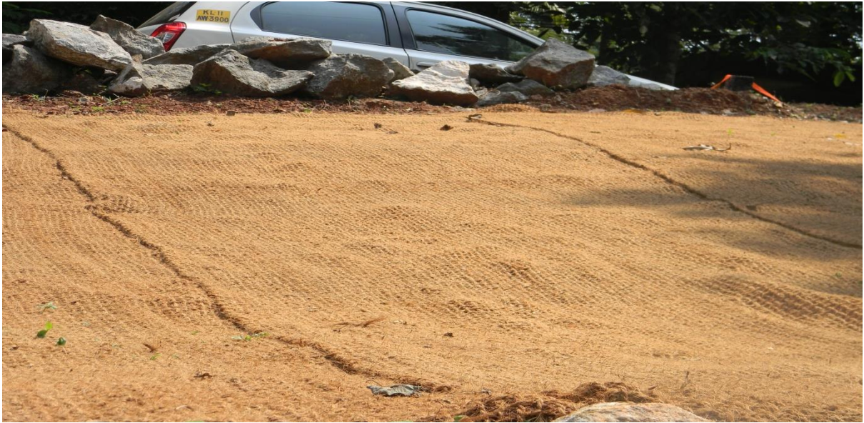
Plate 11. Soil conservation measure using coir geo-textile| in the demonstration plot
